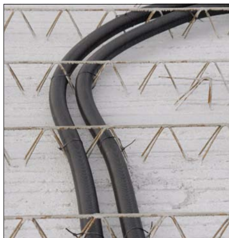
New build Installation in concrete ceiling
