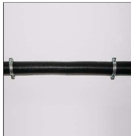
Renovation Installation in false ceiling*
