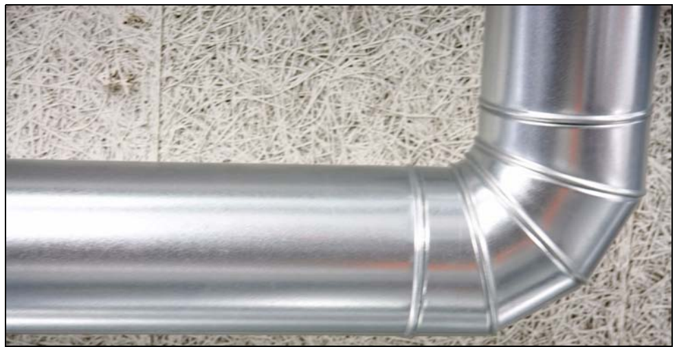
Installation of folded spiral-seams ducts
