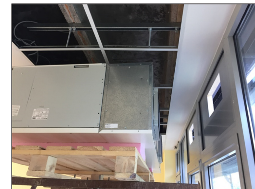
11. Fit the unit (including the mounted terminal box) onto the two designated cut-outs on the façade and screw the façade element to the frame. The sealing strip used provides a sealed connection between the façade element and frame.
